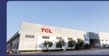
Bulk Parts Factory
